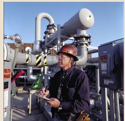
Approximately 3,980 feet of steam pipeline was installed for the DUS project
