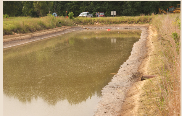
De-watering of the TNX Seepage Basin
