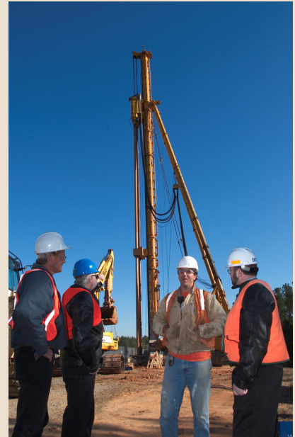
Drill rig used to construct grout columns at F & H Groundwater
