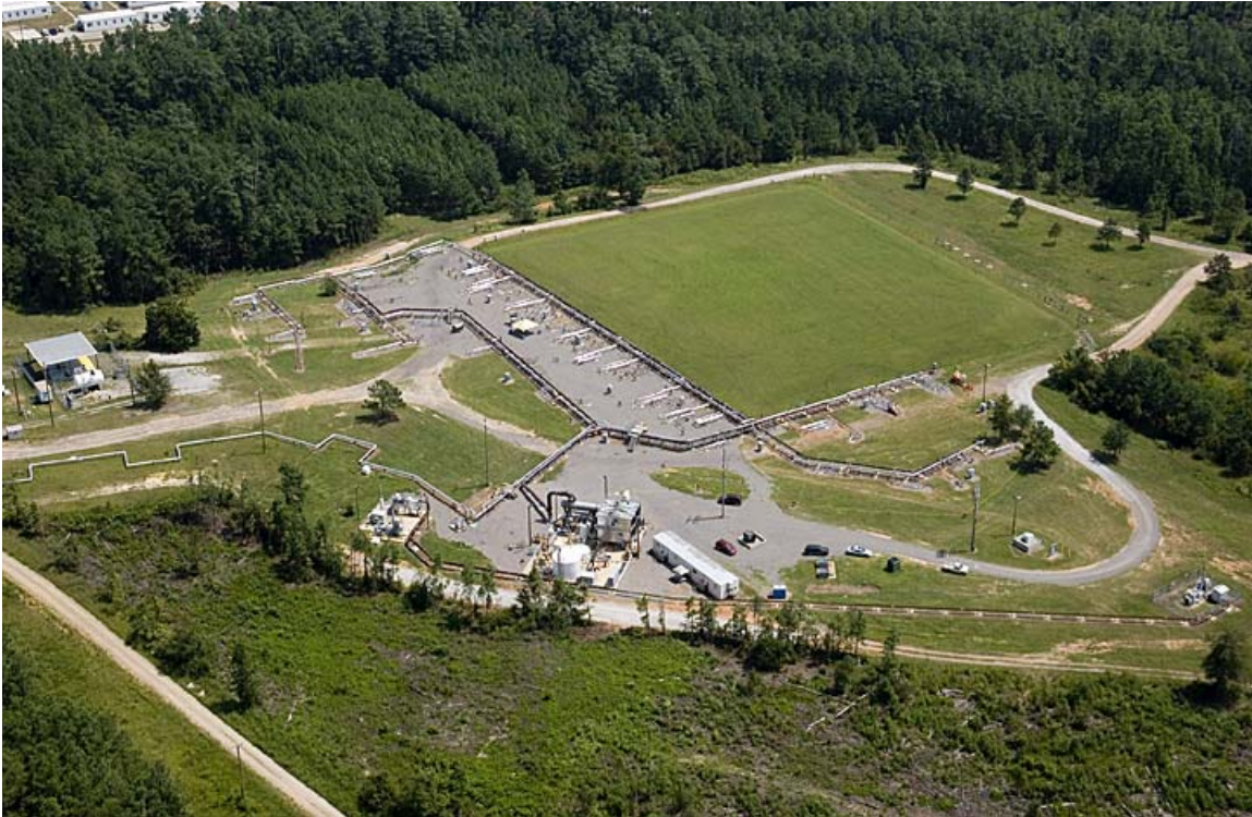
Aerial view of DUS project
