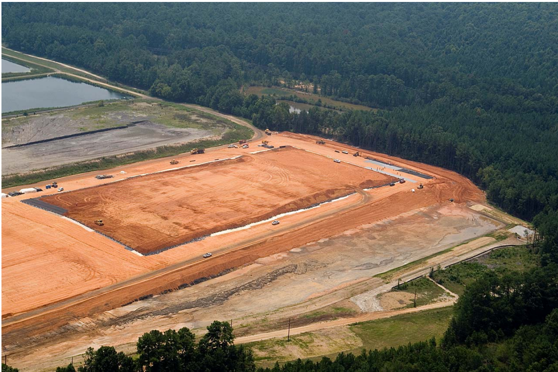
Aerial view of geosynthetic cap construction
