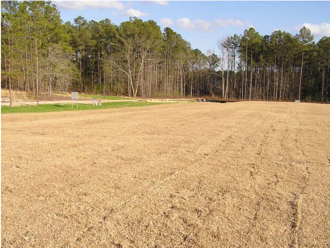
RBRP and RRP after cap construction complete
