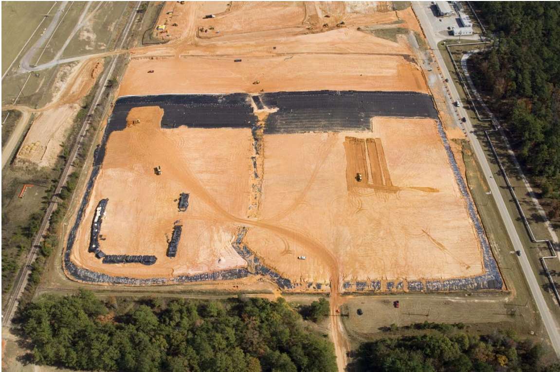
Aerial view of cover construction
