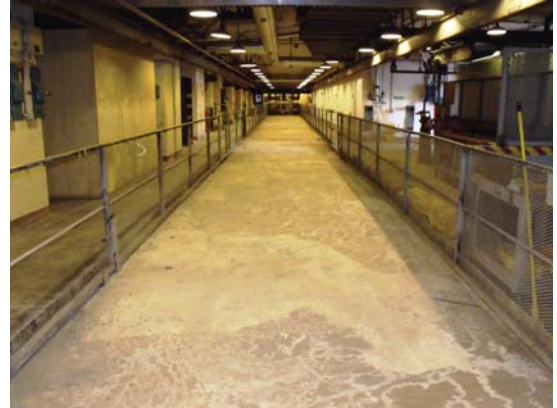
Completed Grouting Activities in C-Reactor Disassembly Basin
