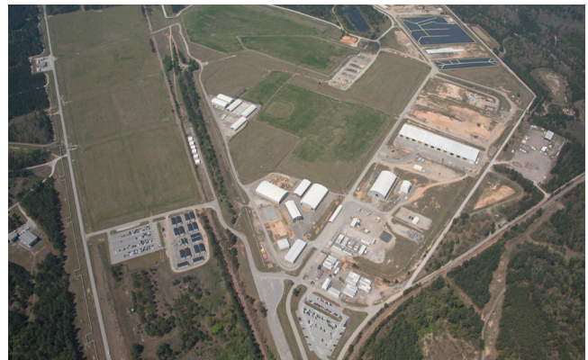
The Solid Waste Management Facility at SRS.
