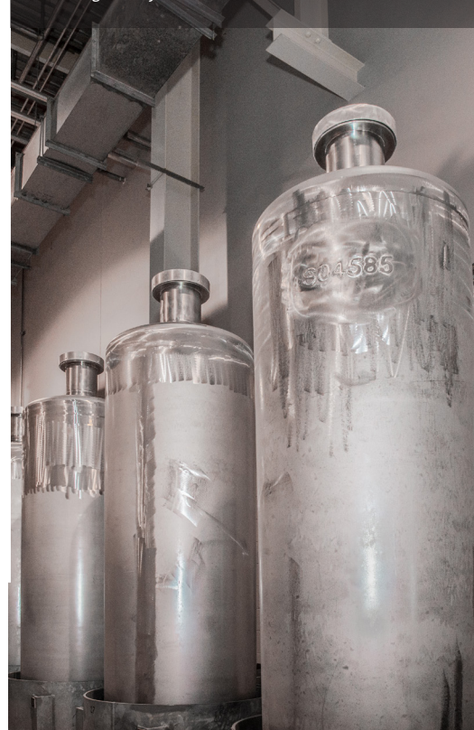
Empty canisters await being used in the Defense Waste Processing Facility
