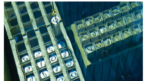
Used nuclear fuel assemblies in L Basin
